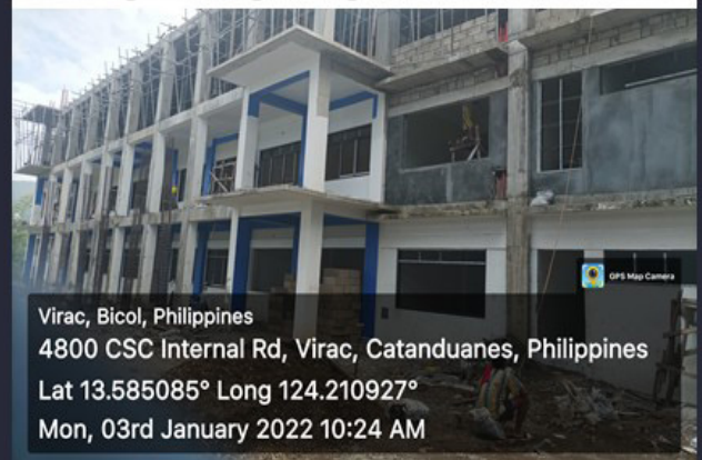
Repair/Rehabilitation/Retrofitting of Laboratory Building of College of Agriculture and Fisheries
