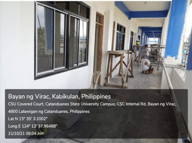
Completion of CAS Academic Building
