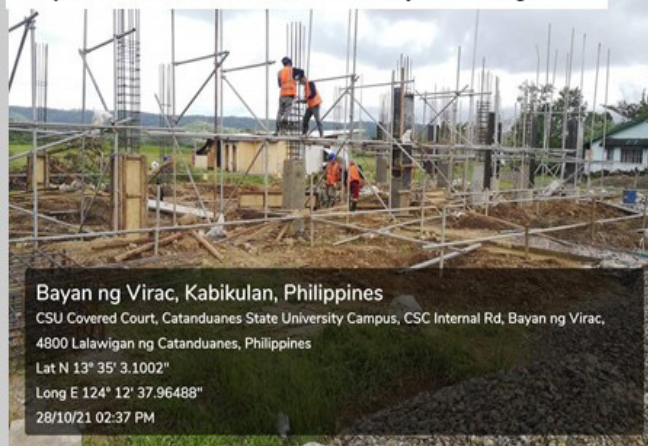
Repair/Rehabilitation/Retrofitting/ Replacement of Food Laboratory Building
