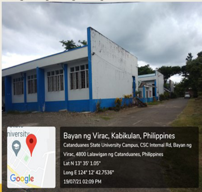
Repair/Rehabilitation/Retrofitting of College of Engineering Building
