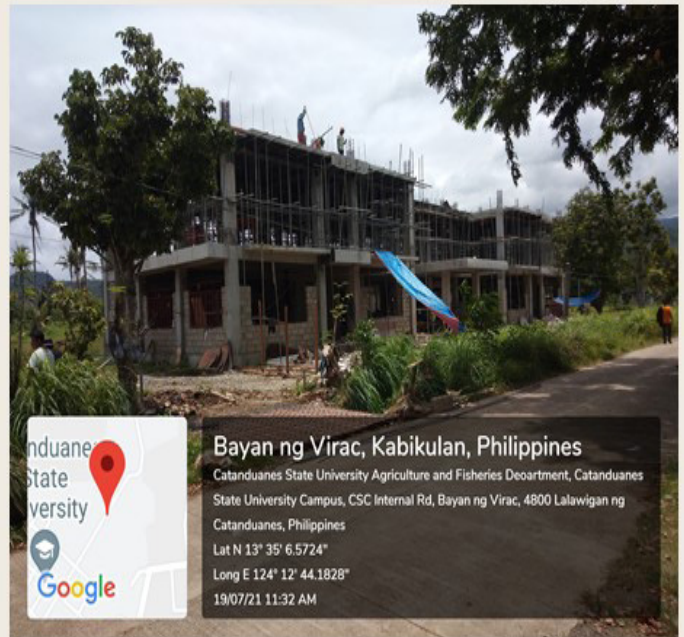
Construction of Men's Dormitory
