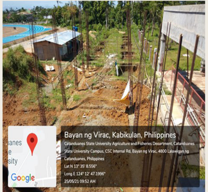
Completion of University Sports & Cultural Center (Grandstand Building B)
