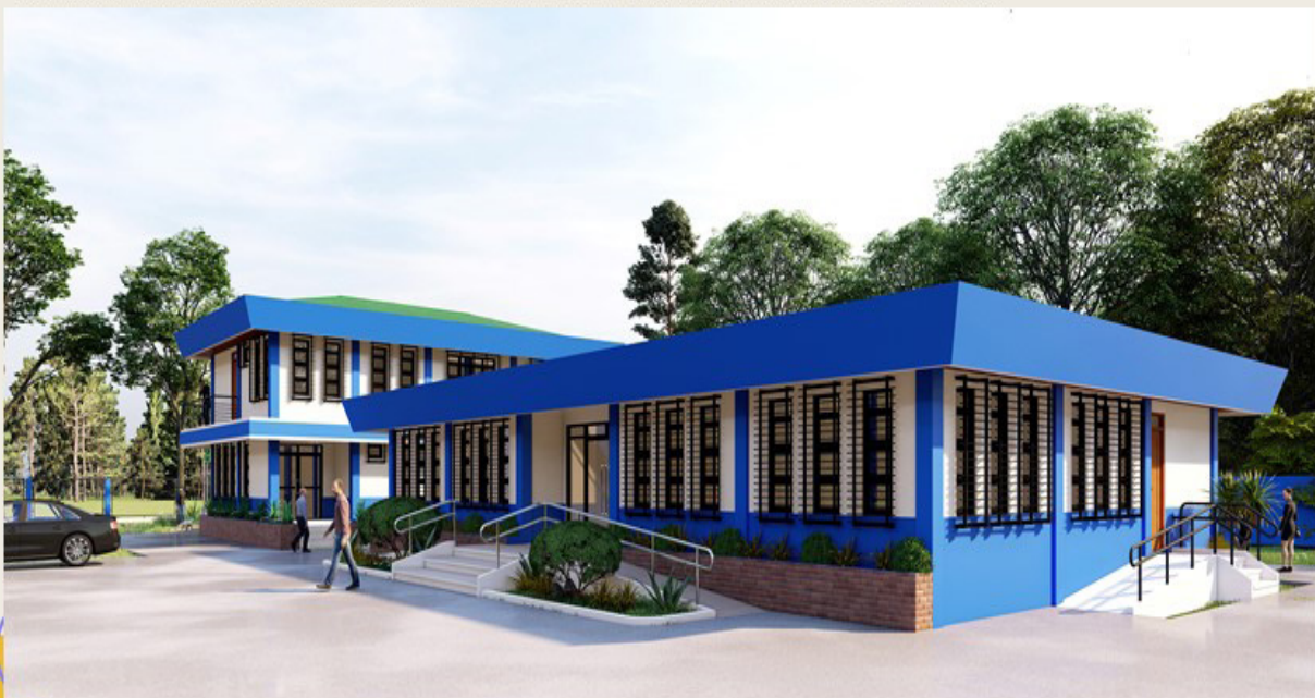
Repair/Rehabilitation/Renovation/Retrofitting of ATIC Building (formerly FIDA Building)
