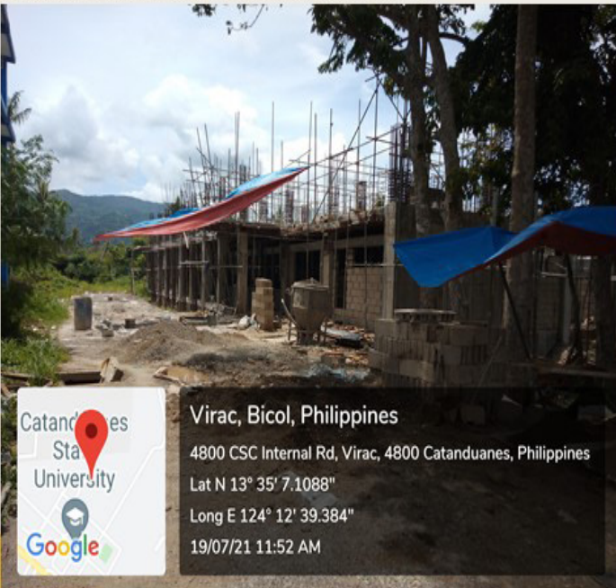
Repair/Rehabilitation/Retrofitting of College of Agriculture and Fisheries Laboratory Building
