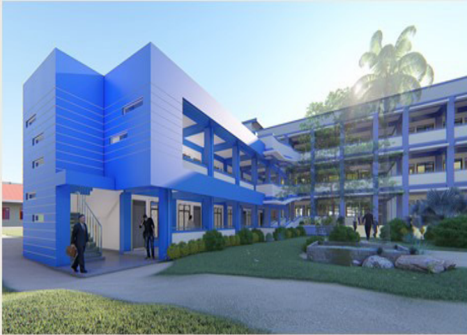
Completion of Technology Building A & B
