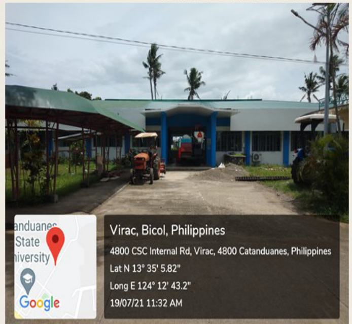
Repair/Rehabilitation/Retrofitting of College of Agriculture and Fisheries Building
