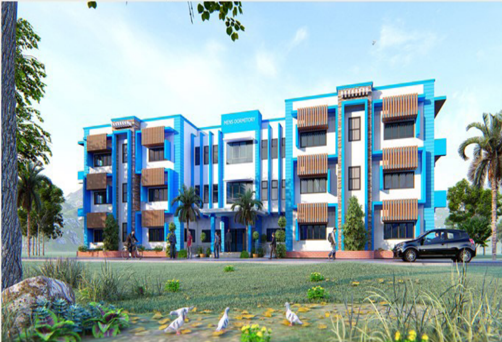
Completion of Men's Dormitory
