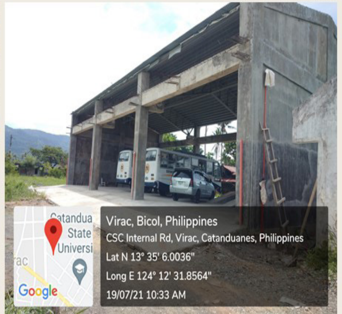
Completion of Buildings and Grounds Services (BGS) Building
