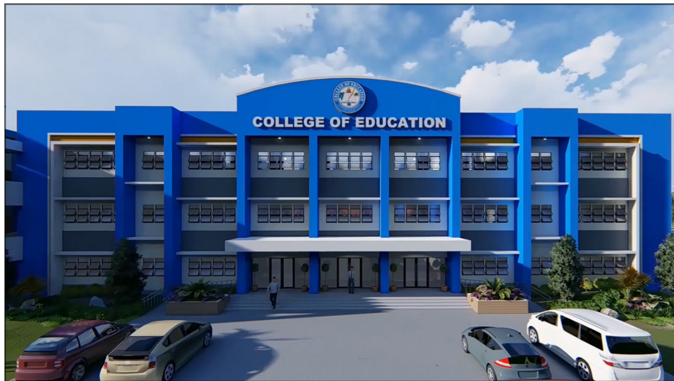
Name of Project: Repair/Rehabilitation/Retrofitting of College of Education Laboratory School Building Project Amount: P100,000,000.00
