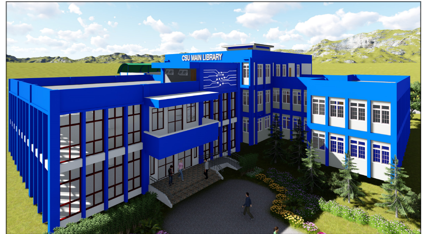
Name of Project: Completion of Main Library (Establishment of e-Library) Project Amount: P15,000,000.00
