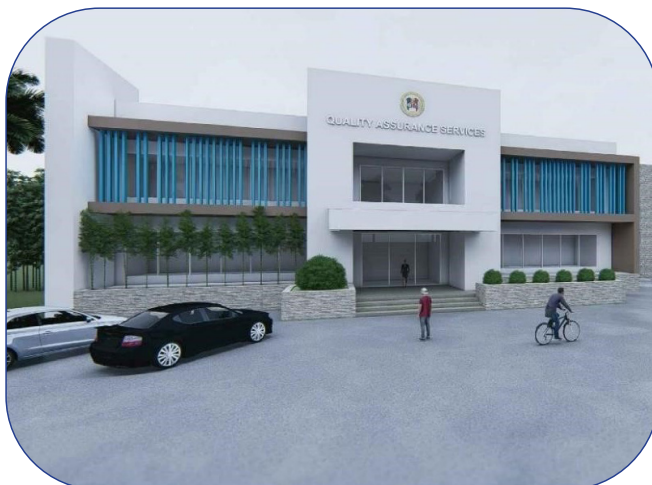
Modernized Quality Assurance Building of the Catanduanes State University
