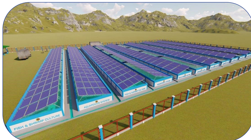
Concrete Fishpond for Fish & Shrimp Culture & Aquaponic System with 518.4 KW Microgrid Solar Power System
