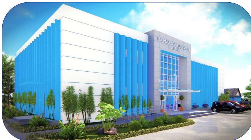
Two-Storey Panganiban Campus Technology Education Building
