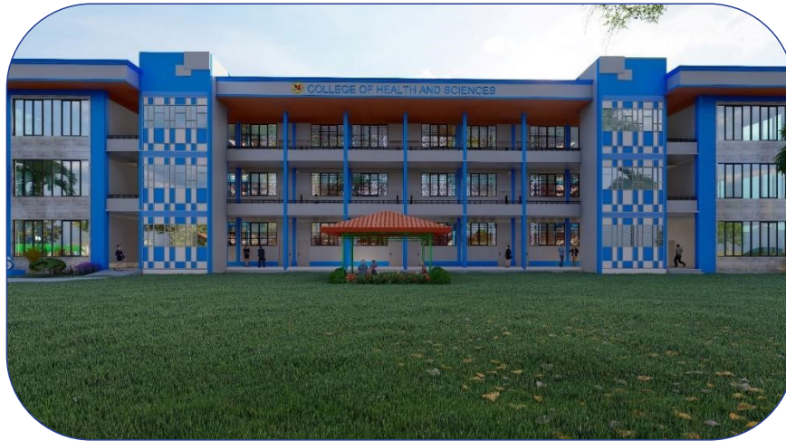
College of Health Sciences Academic Building (Retrofitted/Expanded)
