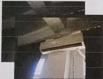
An air-conditioning unit is mounted on the wall of the room to maintain the optimal temperature for the maintenance of computers
