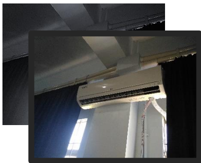
An air-conditioning unit is mounted on the wall of the room to maintain the optimal temperature for the maintenance of computers
